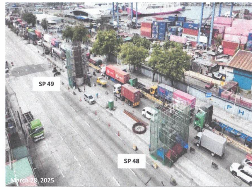
SP 48 & SP 49 Rebar installation in preparation for column works
